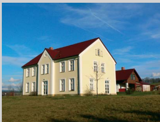
Family house, farm country house - boiler-room is placed in a separated, sole farm building incl. other rear areas (carport, workshops, cellar)
