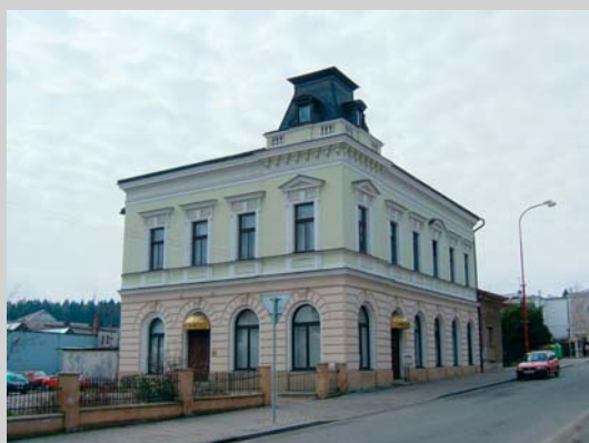
Office building - boiler-room is situated downstairs, however boiler-rooms were realized even in the attic in case of similar buildings
