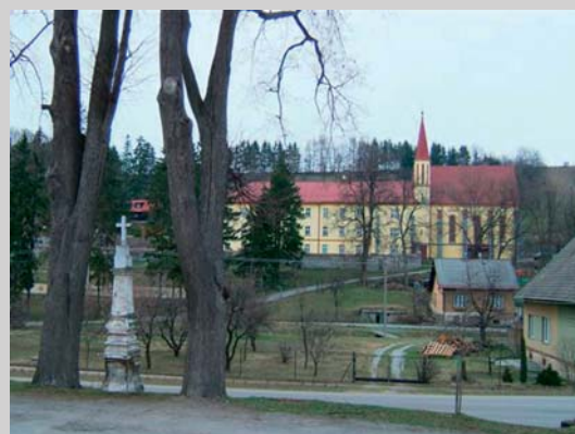
Monastery incl. chapel - in this monastery the heat pump was replaced by VERNER boilers cascade placed in the neighbouring building
