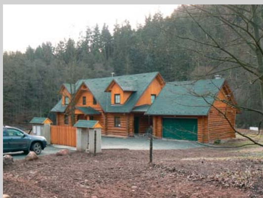
Wood log house - boiler-room (incl. fuel storage) is situated in the shared united building with garage.
